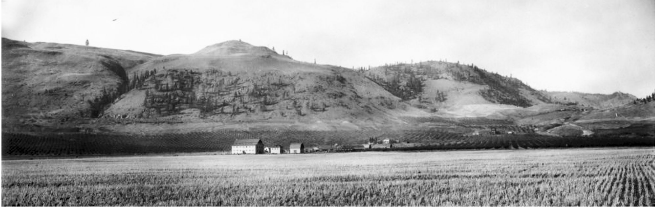
Community fruit packing house (far left) and other industrial buildings near Carson, circa 1928. Village No. 6 (Gritchin Village), Spencer Hill, and Hardy Mountain can be seen in the background.
