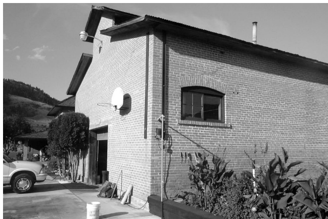
Jam factory boiler house as it appeared in 2002.
